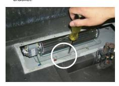
12) Pull Fan Assembly forward, to disenagage the fan clip on the rear wall. Then lift the Fan Assembly up and pull through firebox opening.
